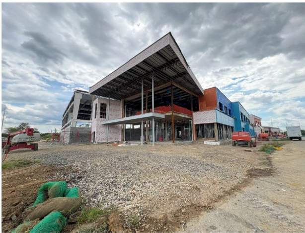
09/05/25 – Exterior – Northwest Corner
