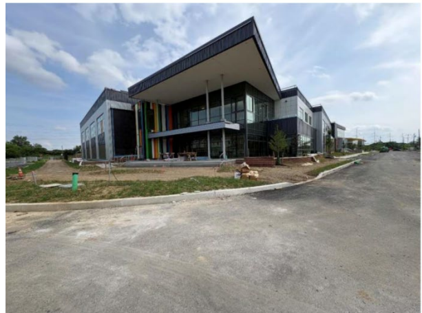
06/10/26 – Exterior – Northwest Corner
