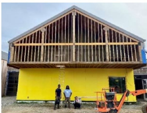
Trainees working on the façade
