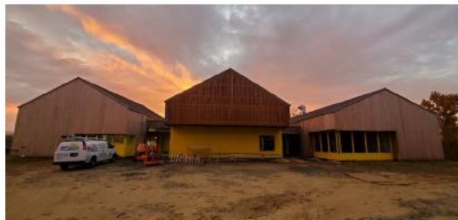
Completed façade, December 2023
