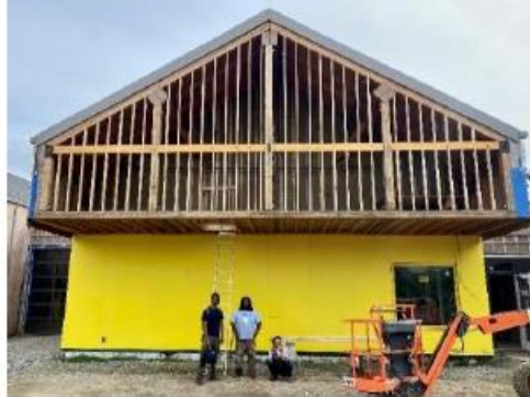
Trainees working on the façade
